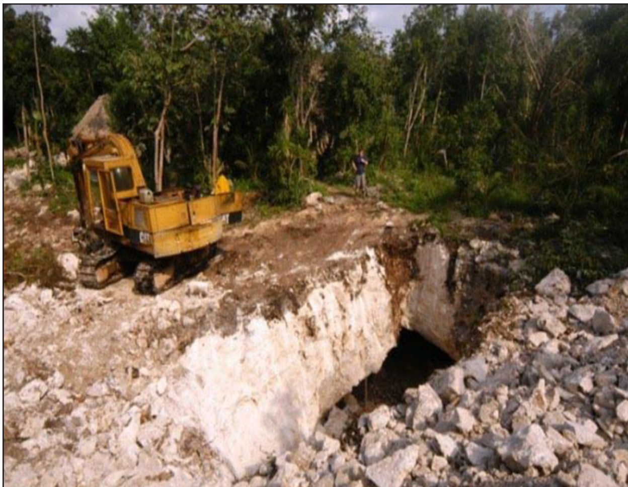
Figure 2 Recent example of cenote enlargement using heavy machinery. The landowner created an open water pool to attract paying snorkelers. (Photo by Robbie Schmittner)
